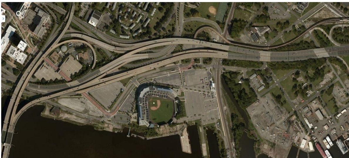
Figure III.20 I-264 and the Berkley Bridge near Harbor Park and Tidewater Gardens
