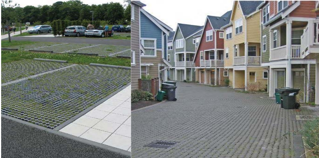
Figure IV.2.5 and Figure IV.2.6 Example of Permeable Pavers
