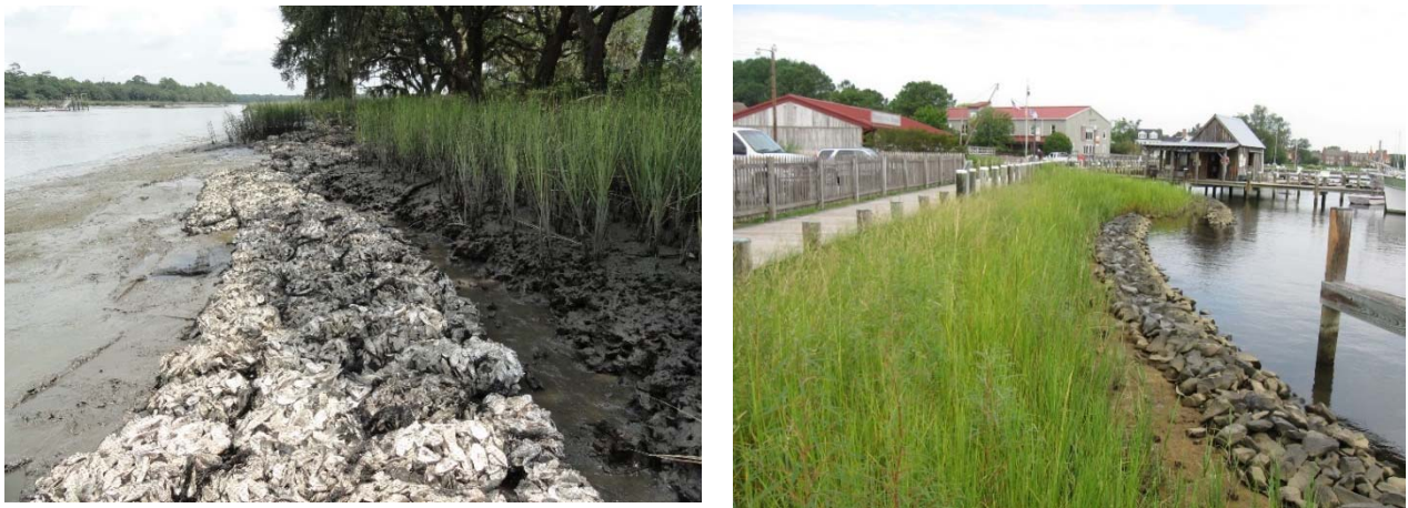
Figure II.19 Examples of Living Shorelines with Protective Sills (oyster shell on left, stone on right)
