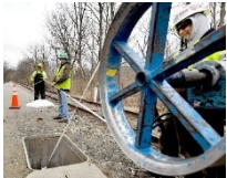
Broadband work in York County, VA
