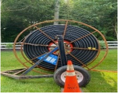
Broadband work in James City County, VA
