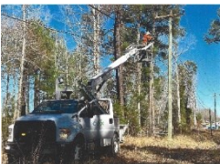
Broadband work in New Kent County, VA
