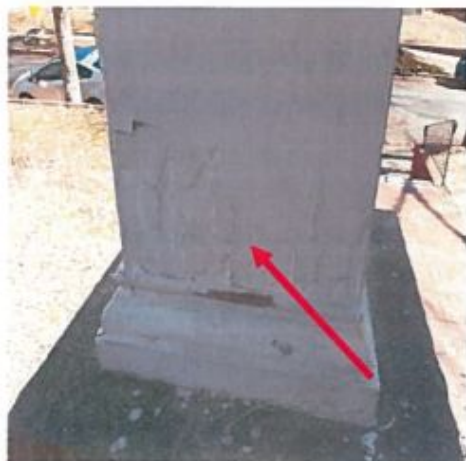
Photo 7: Front porch column post and column base (corner AD) with identified deteriorated LBP.
