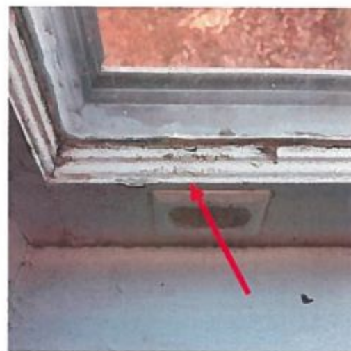
Photo 15: Window 6, window trim and window sill (side B) in dining room with identified deteriorated LBP.
