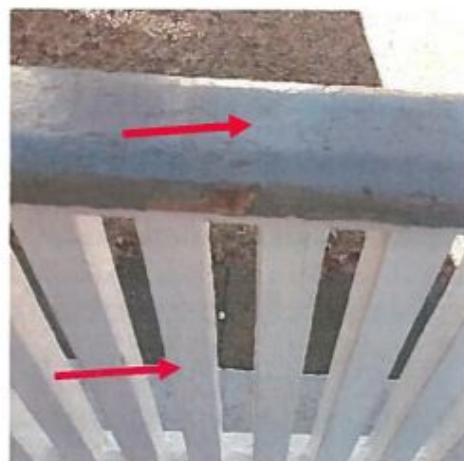
Photo 8: Front porch rail cap and balusters with identified deteriorated LBP.
