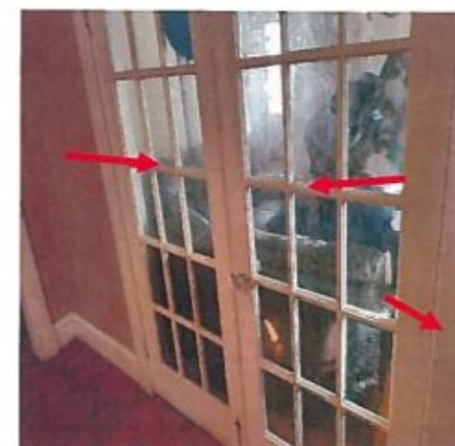
Photo 14: French doors and door trim in dining room (side A) with identified deteriorated LBP.
