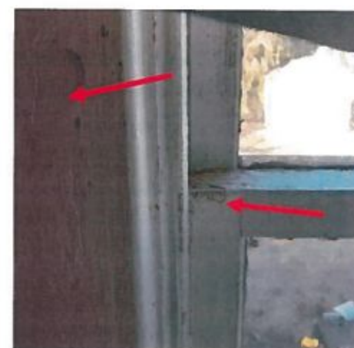
Photo 16: Window 7 and window trim in dining room (side C) with identified deteriorated LBP.
