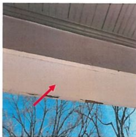
Photo 6: View front porch ceiling beam (side A) with deteriorated lead-based paint (LBP).
