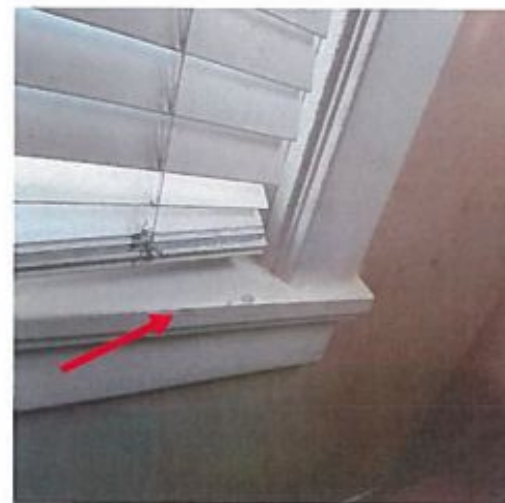
Photo 13: Window 3, trim and sill in living room (side A) with identified deteriorated LBP.
