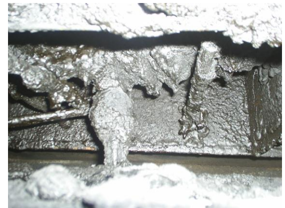
Plenum area of a hood. The fire-extinguishing system link and nozzle are covered with grease from Asian cooking.
