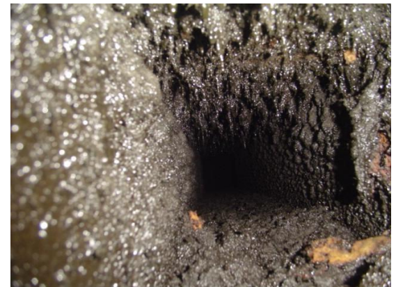
Grease accumulation from gas char broiler (predominantly hamburger cooking) in a horizontal section of ducting
