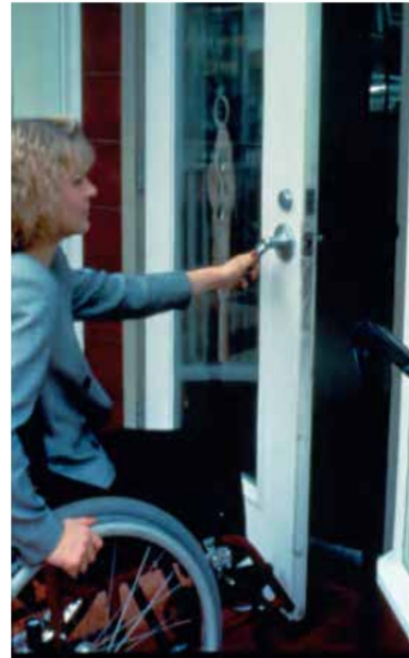
Changing hardware is a low-impact means to help create accessibility to historic buildings.
