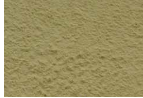
Detail showing texture of stucco above. Right, stucco applied to the upper floor of a downtown commercial building.
