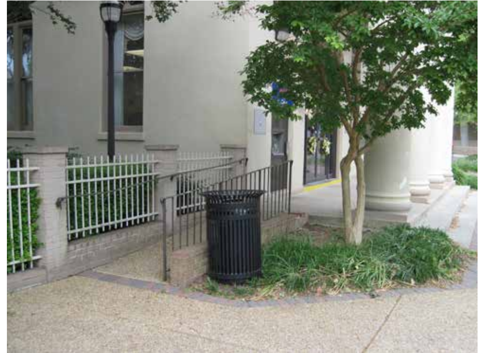
A handicap ramp example in Gloucester, Virginia that carefully works with the topography without negatively impacting the historic building.
