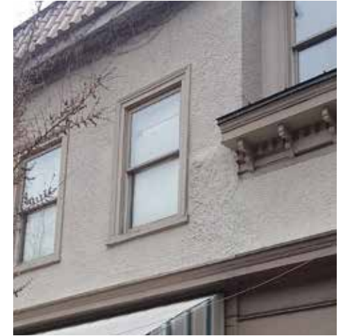
Detail showing texture of stucco above. Right, stucco applied to the upper floor of a downtown commercial building.
