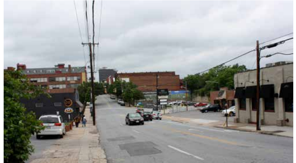
Example of streetscape issues including failing sidewalks and street paving.
