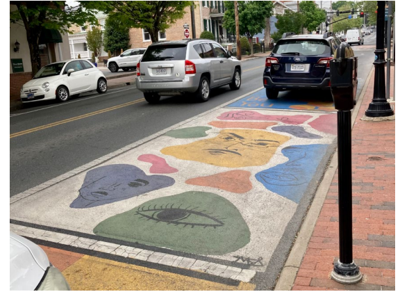
City of Winchester's Streetscape Improvement Project
