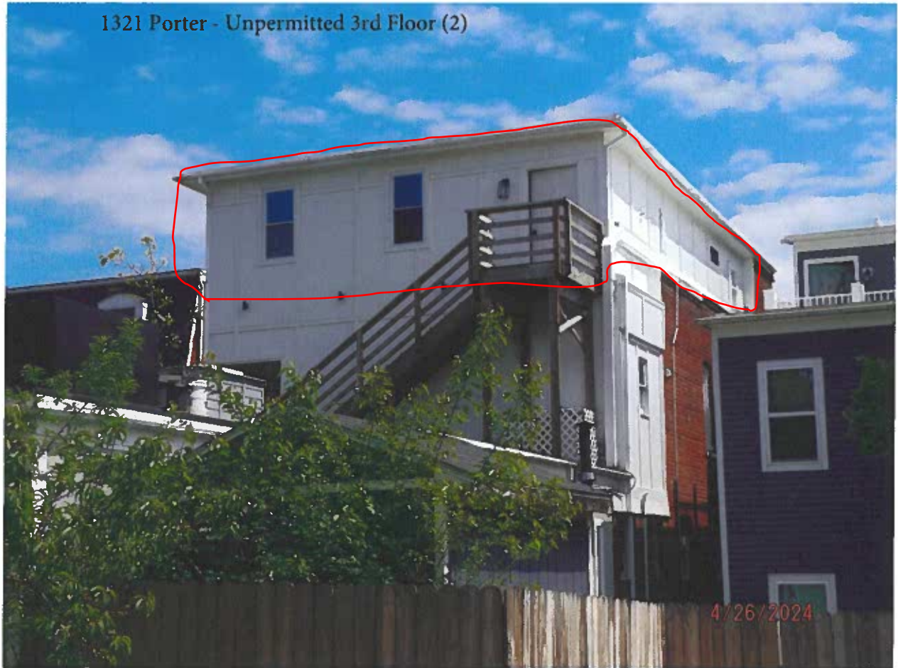
Pictures were taken by Walter Jackson Property Maintenance Inspector
