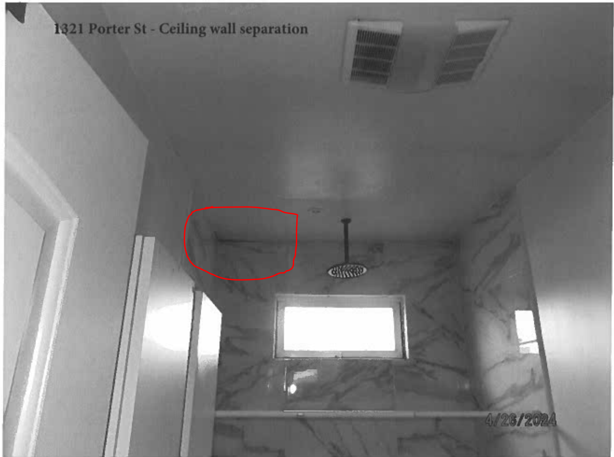
Ceiling/wall separation within 3rd floor addition structural work concealed.
