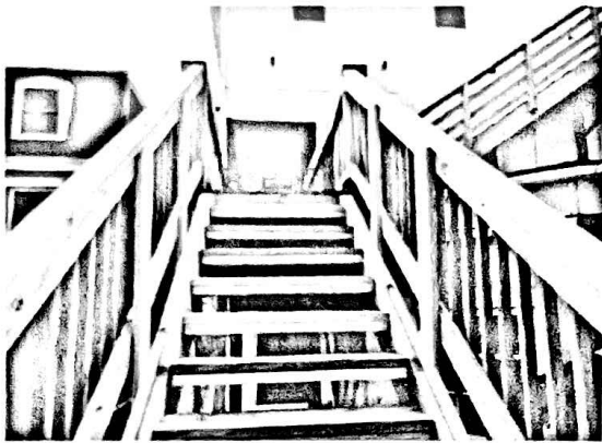
Photo #4 – Additional stringers and treads added. Newel post to be replaced with 4 x 4 posts per attached drawing.
