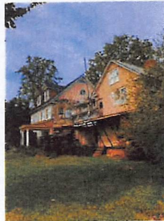
(Picture 3: Shows faulty structural supports, Inadequate roofing on right side, wood rot, and peeling paint)
