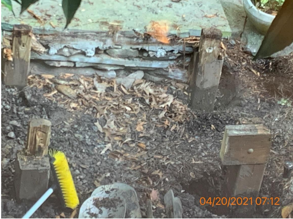
Figure 3- Demo photo of original deck posts
