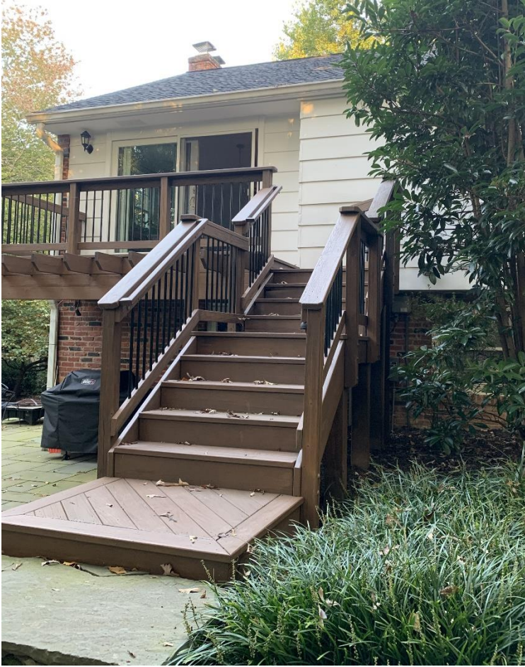
Figure 23 - Another angle of original deck stairs for context
