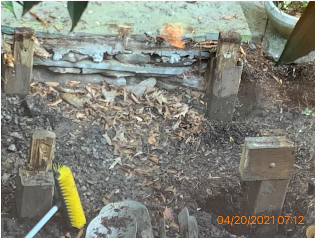
Figure 3- Demo photo of original deck posts
