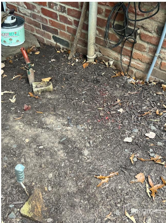
Figure 4 - Original cut down post photos location under upper right landing where new deck was attached to cantilever
