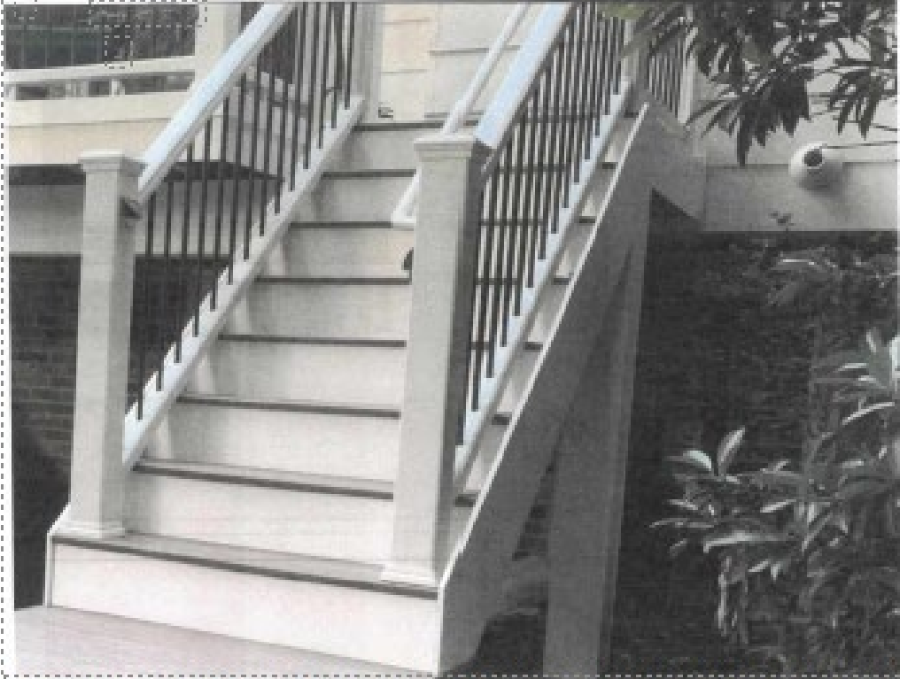
rails were installed directly to the balusters/downhand of the frame which is prohibited. The prior installed deck design that was requested to be followed had separate support and posts installed under the stairs which the contractor cut down to the ground. Reference I 1 listed inspections failure items.
