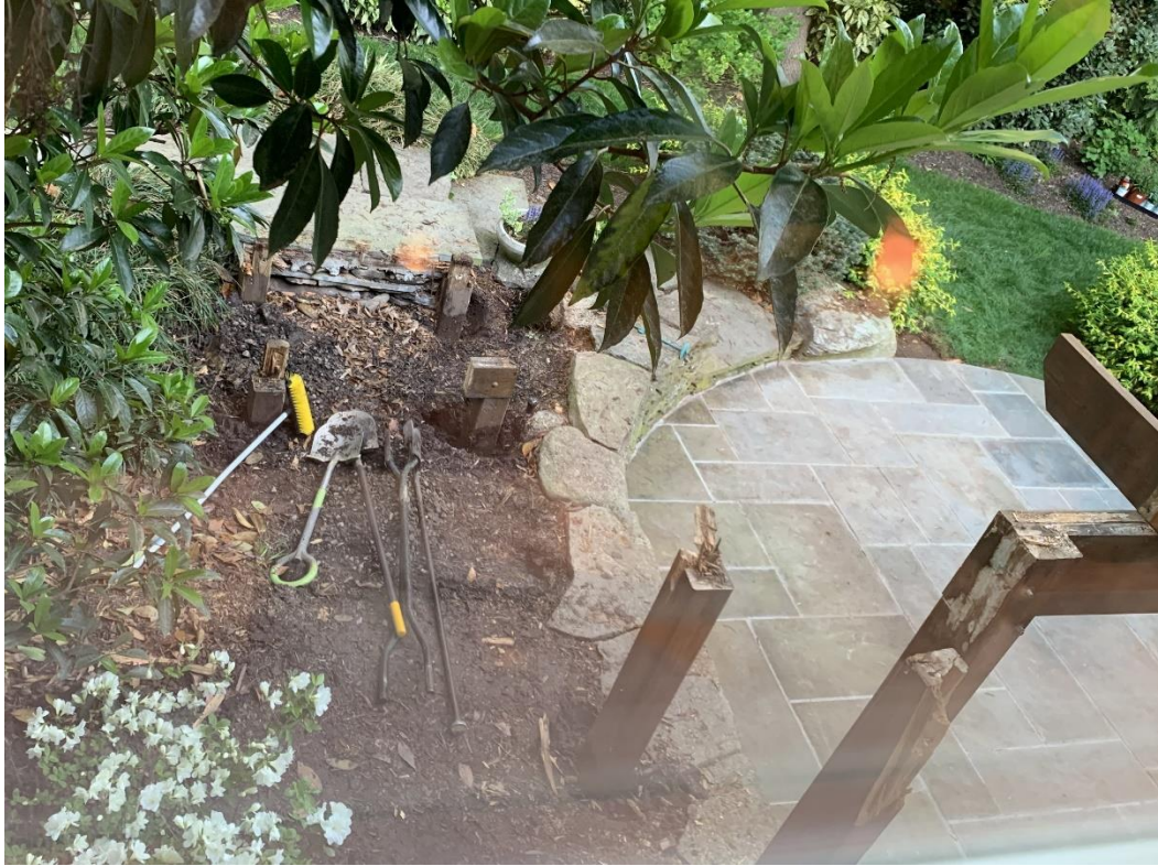
Figure 2 - Demo photo showing removal of original deck stairs posts
