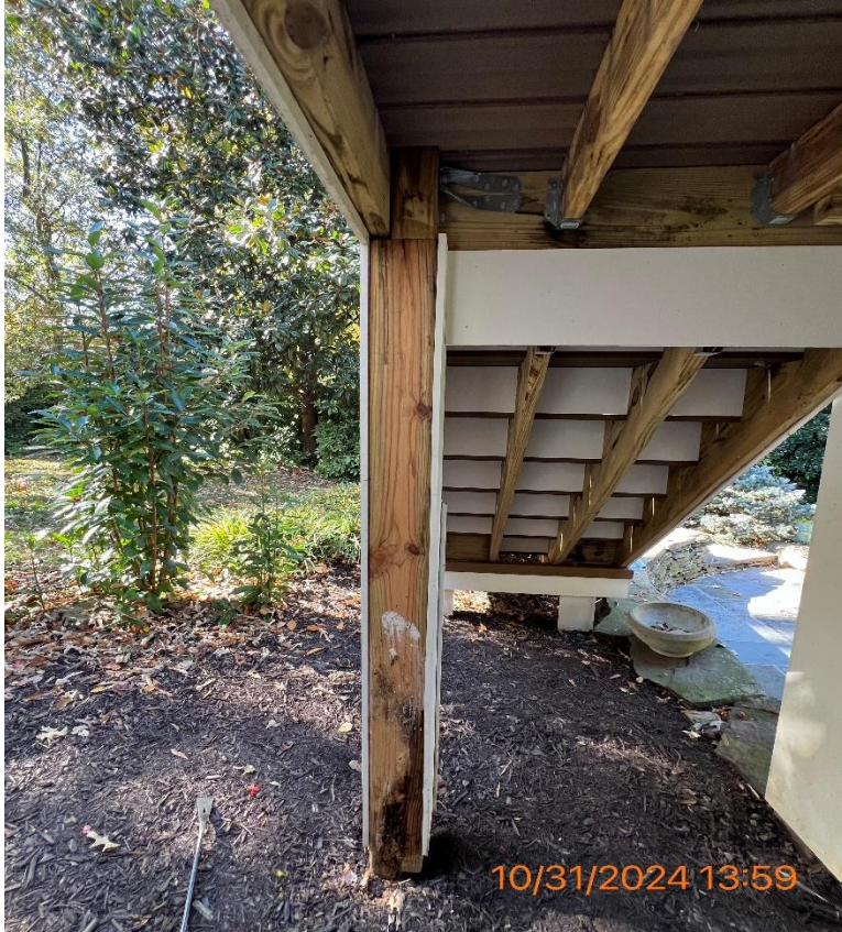
Figure 6 - Full view of incorrectly notched post with PVC removed and post to beam connection pg 14 _ figure 18
