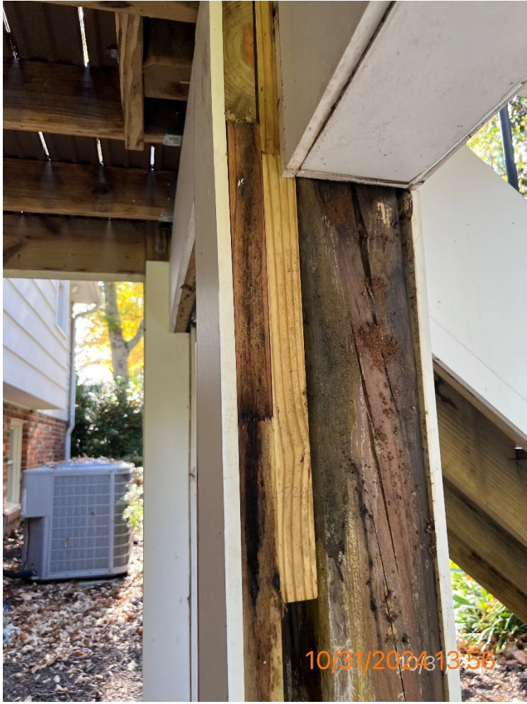
Figure 13 - Another snapshot of altered existing post
