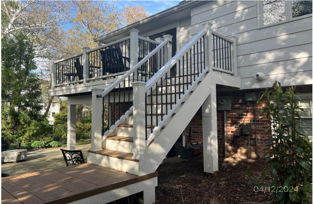
Figure 1 - Full Deck View built by GLK Construction Services Inc.
