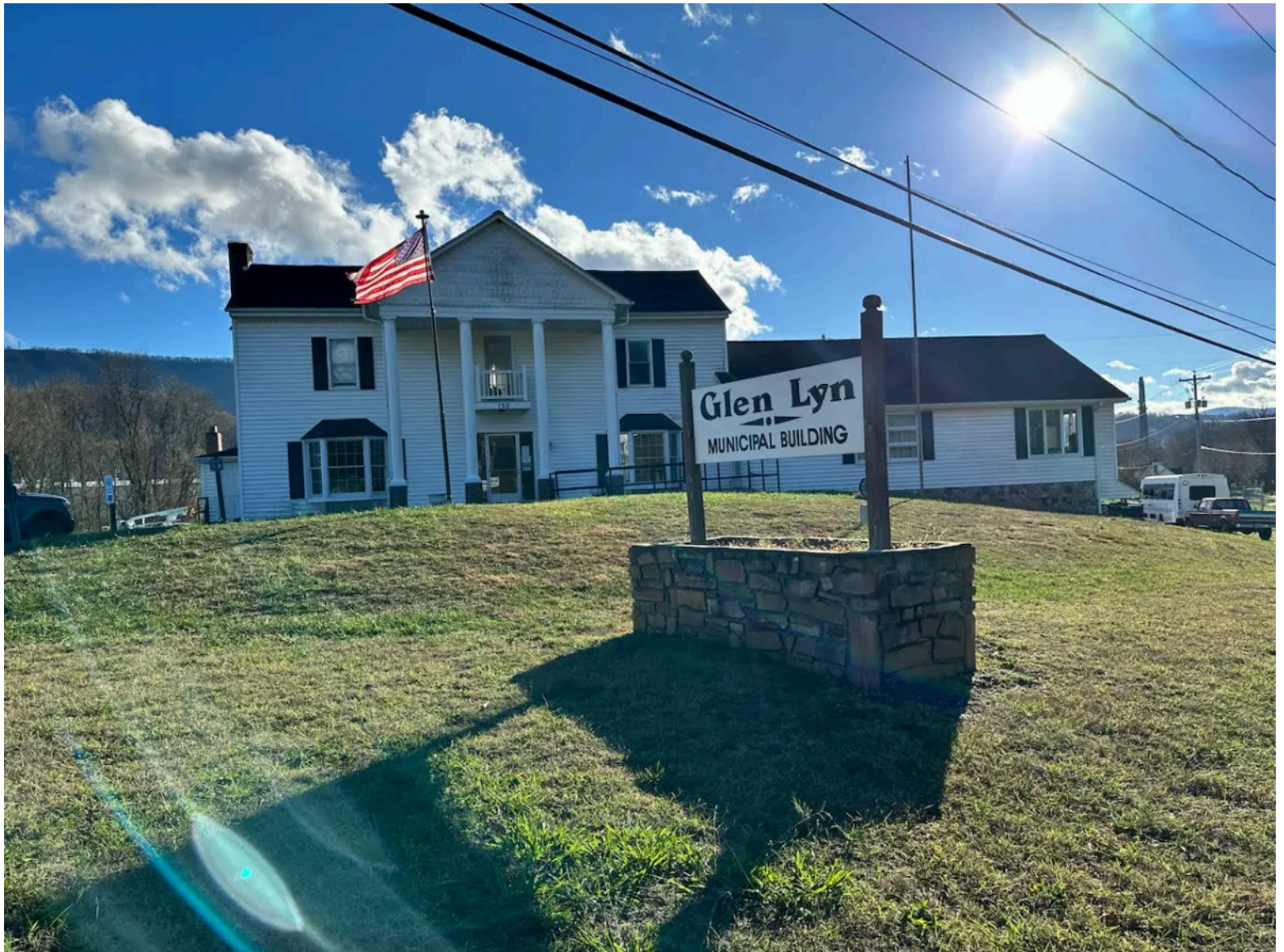
Glen Lyn municipal building. Photo by Michael Hemphill.
