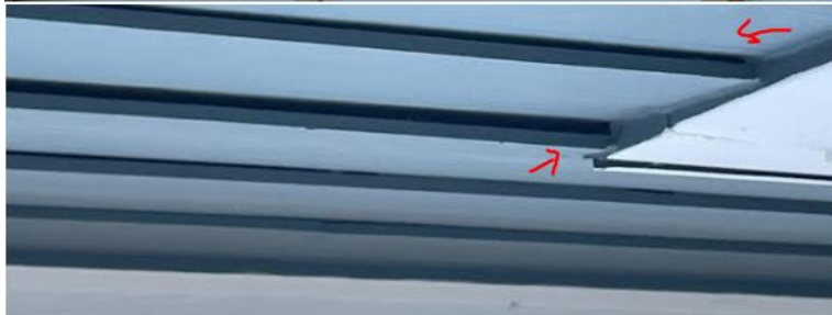
These photos taken by Lisa Gearhart on 12.15.2023 Appeal No 23-10 Violation: Exterior Concrete Lap Siding R703.10.2
