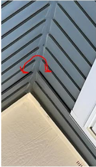
These photos taken by Lisa Gearhart on 12.15.2023 Appeal No 23-10 Violation: Exterior Concrete Lap Siding R703.10.2
