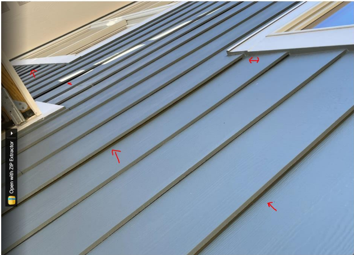
These photos taken by Lisa Gearhart on 12.15.2023 Appeal No 23-10 Violation: Exterior Concrete Lap Siding R703.10.2
