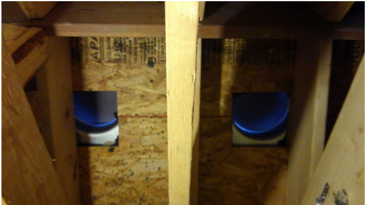
Image 7, Showing 2 of the 8 vents installed in the hip roof.
