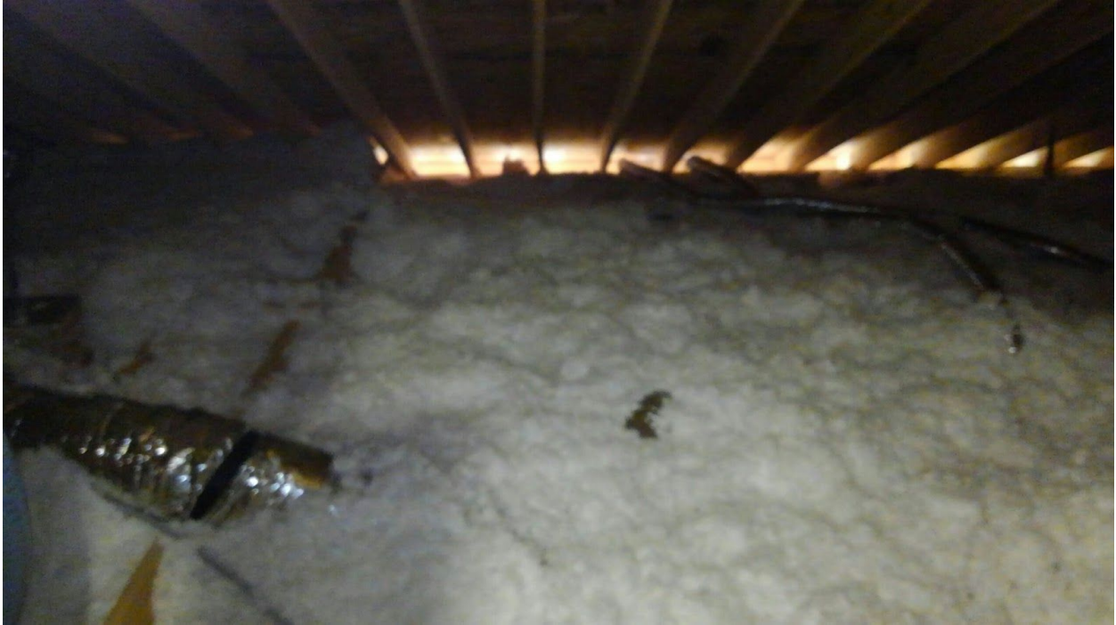
Image 8, Showing Soffit Vents.
