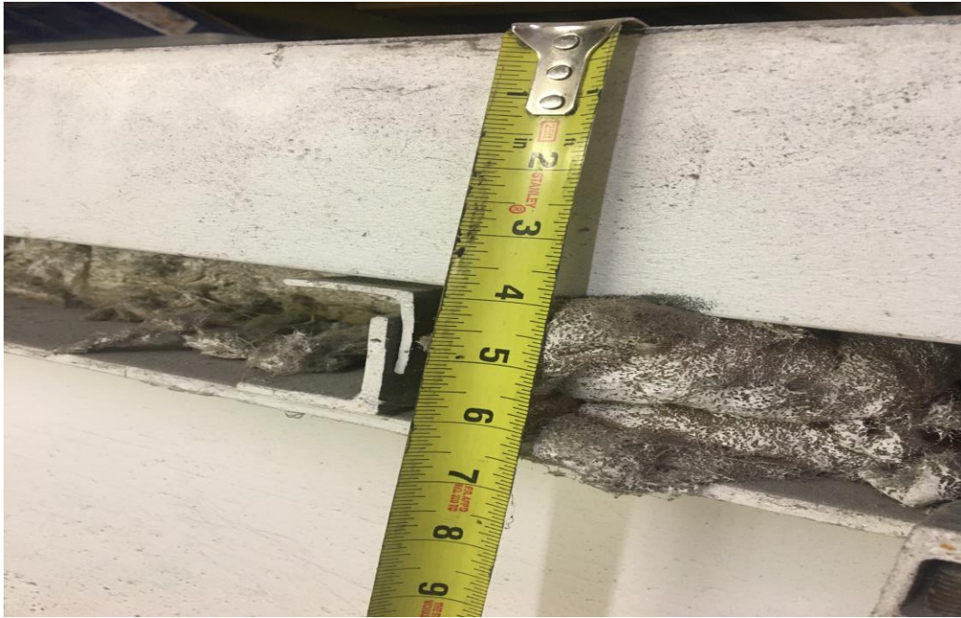
Poured Concrete Thickness
