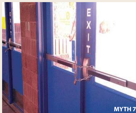
Photo courtesy of Wayne Ficklin
